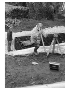
Rainwater soak-away works
